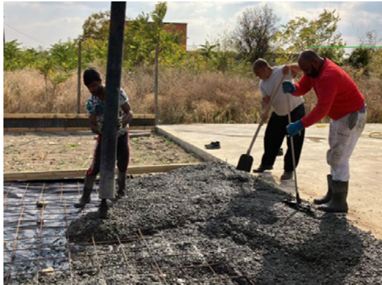
Floor slab of a private house
